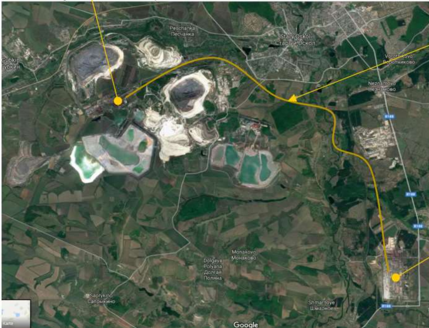
Lebedinskiy GOK, PSP Pump Plant
