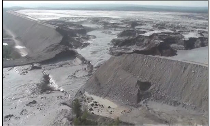
Mt. Polley Tailings Dam Failure in BC
