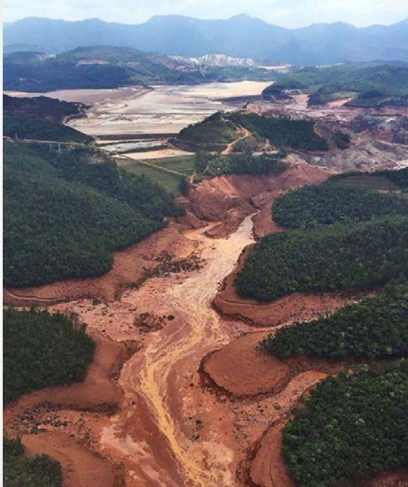
Samarco Dam Failure in Brazil
