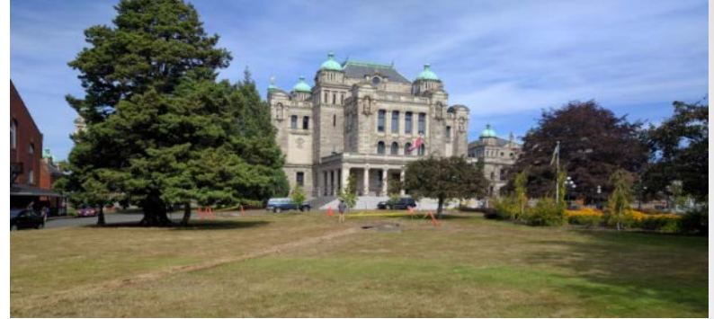
BC Legislature EEWS installed in 2016.
