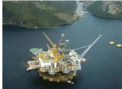
Structural Monitoring System for Offshore Platforms
