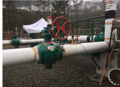
Pipeline Vibration Monitoring in NE B.C.
