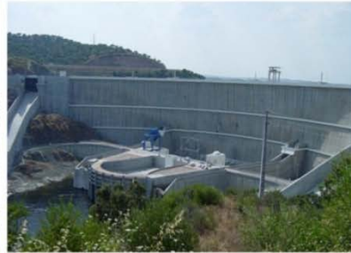
Integrated Monitoring Systems for Dams
