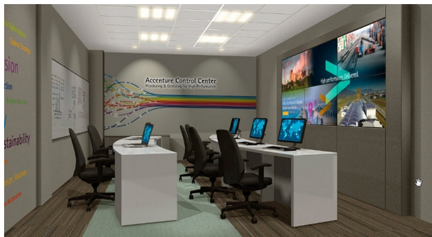
Figure 3 – Example of a remote process control centre
