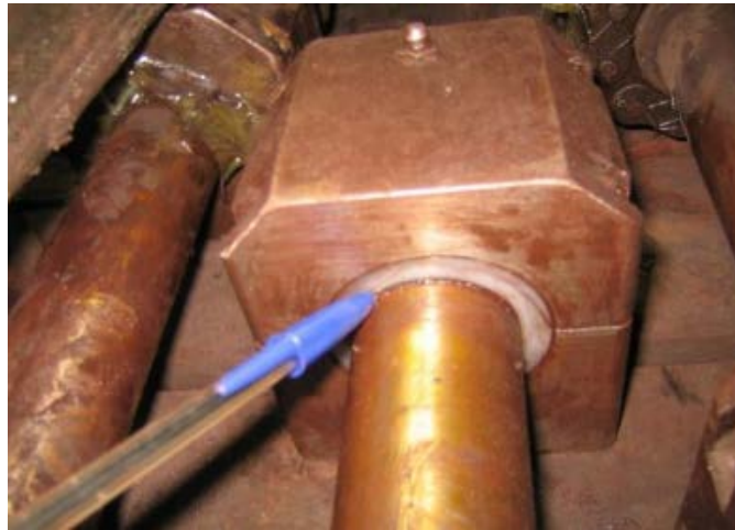
Figure 3: Later surface preparation and sealing, ready to apply the polymer.
