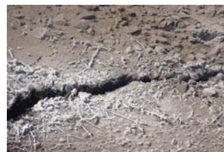
(b) cracks at sampling site
