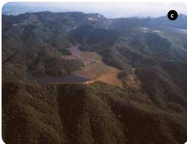
Photo 10 (a, b, c). Dams in mining sites (Source: MBR).
