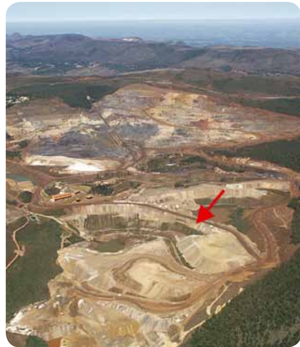
Photo 13. Waste dump under construction downstream from the mine pit. Source: MBR
