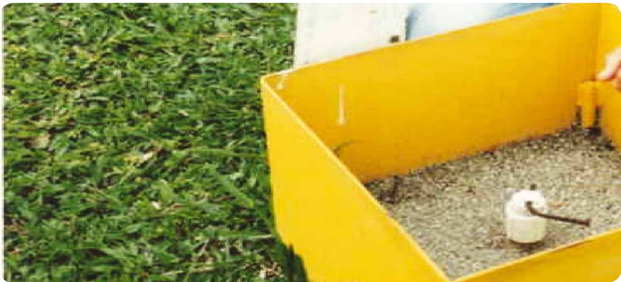
Photo 50: Piezometers in detail
