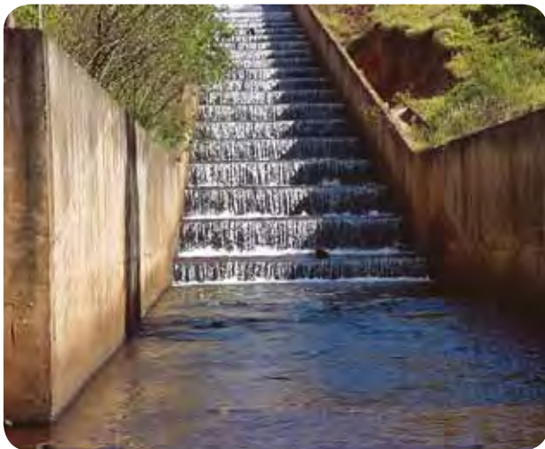
Photo 12. Disposal of dam effluents through a weir. Source: MBR
