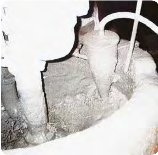
Photo 53. Abrasive sludge pumping tank
