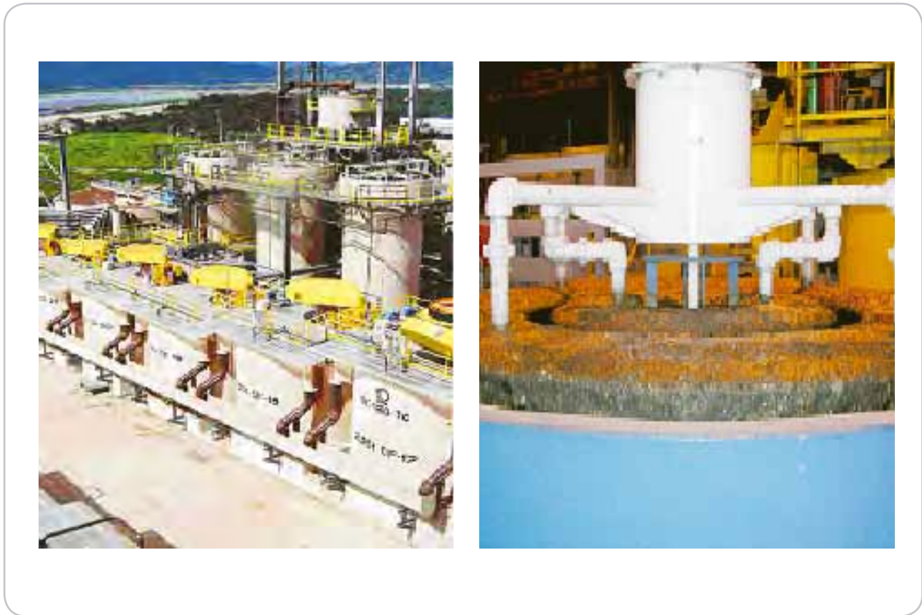
Photo 21. Mechanical and column flotation cells on the right, with the tailings dam in the background, and with foams in the flotation column on the left, Sossego copper plant/mine, CVRD.
