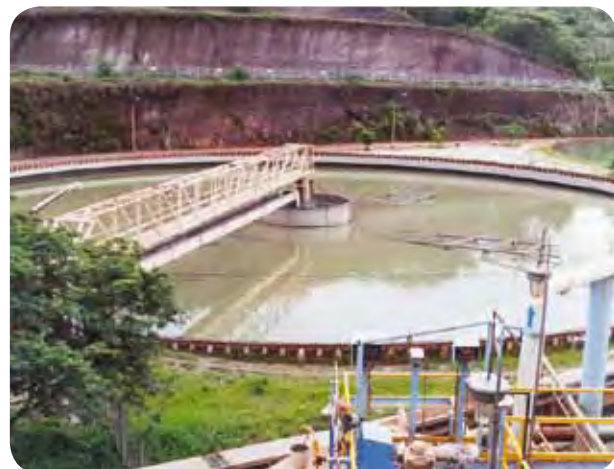
Photo 25. Thickening of flotation tailings in an ore processing plant
