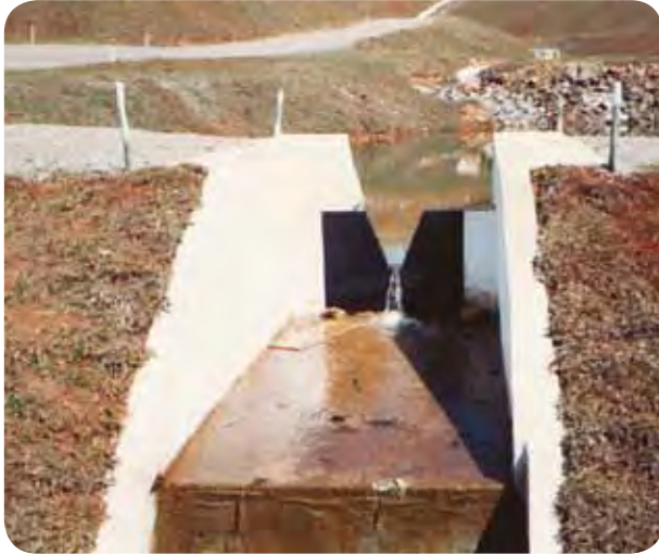
Photo 11. Water drainage through an internal drain in the bulk of the dam. Source: MBR
