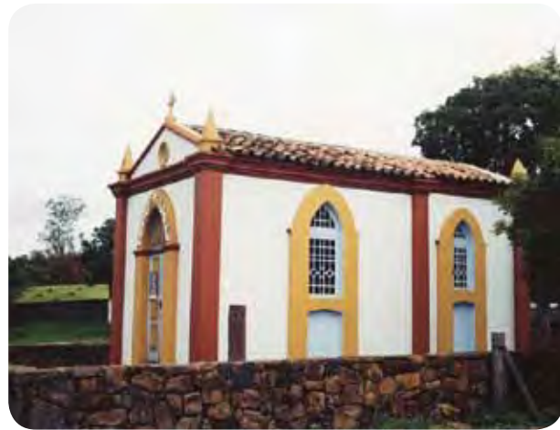
Photo 40. Santa Ana Church after a company-sponsored refurbishment
