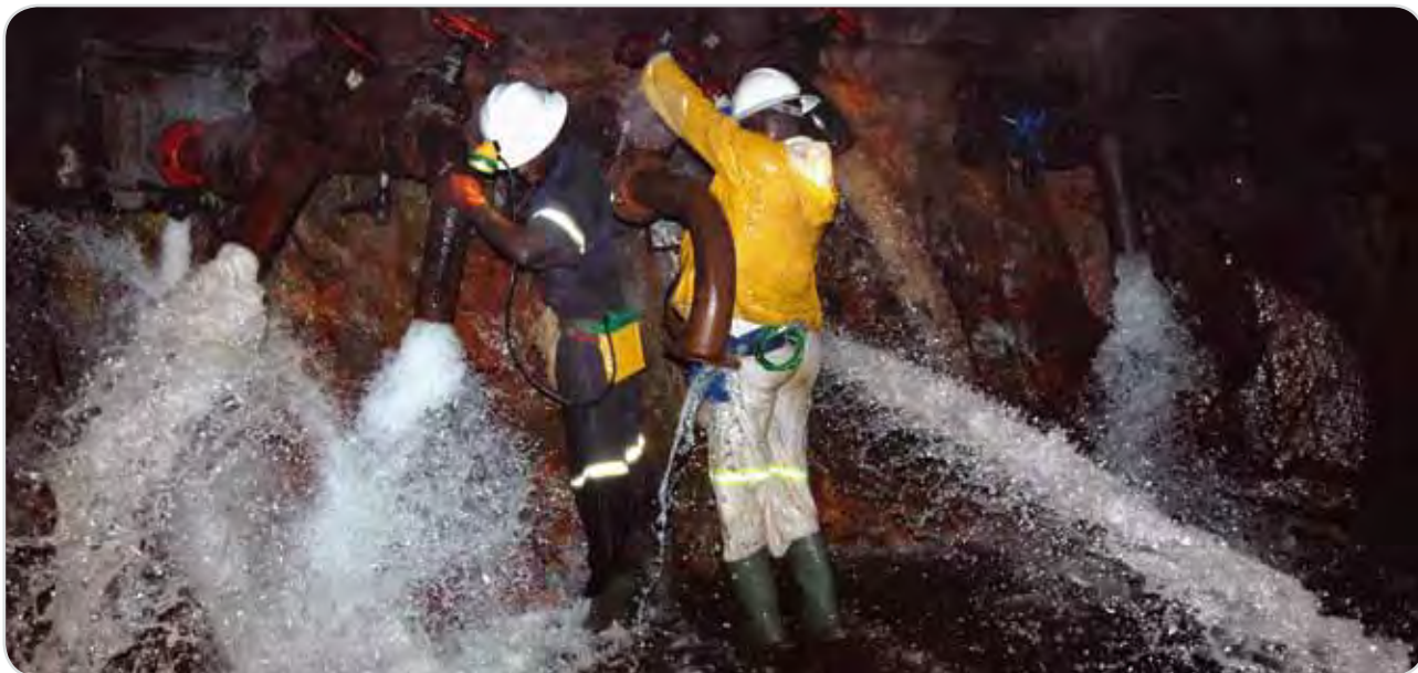
Photo 3. Drainage based on sub-horizontal surveys in a gallery front at the Konkola underground copper mine (Zambia), Konkola Copper Mine
