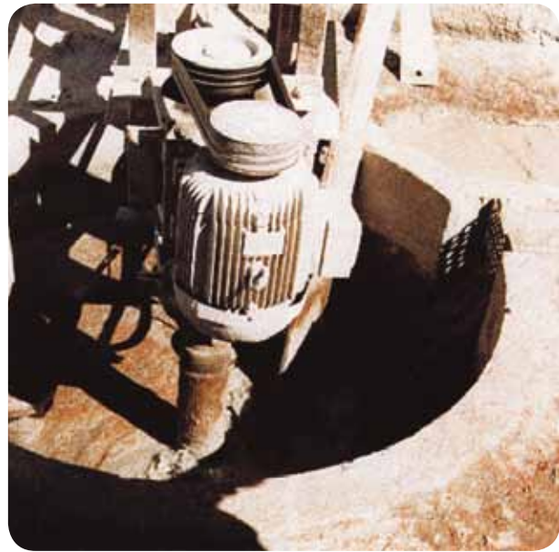
Photo 56. Waste pumping pit for final disposal
