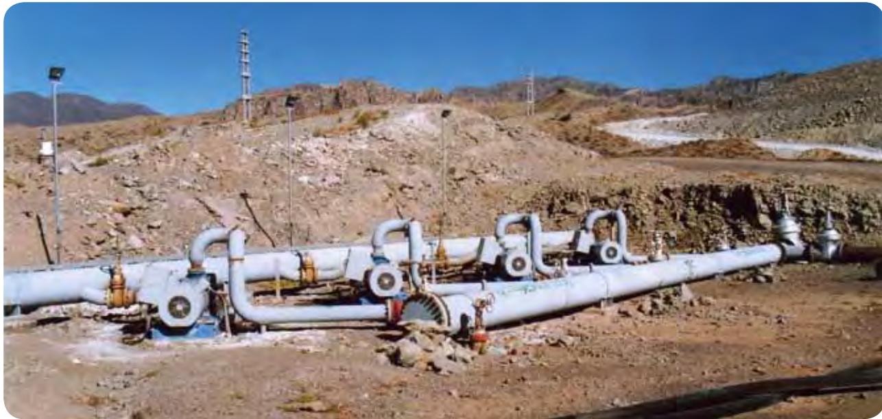
Photo 6. Installation of drainage works at the Bajo de La Alumbrera mine (Catamarca, Argentina)
