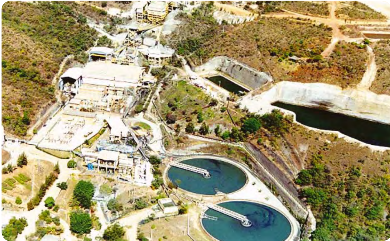
Photo 70. Aerial view of the RPM's processing and hydrometallurgy plant
