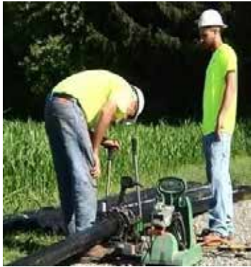
Figure 3: Example of butt fusion
