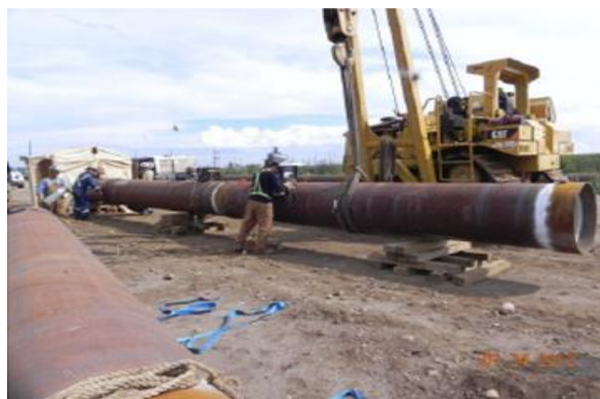
Figure 4: Installation of internally coated pipes at oil sands hydrotransport line
