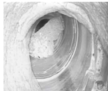
(b) surface vertical well blockage
