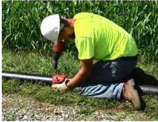
Figure 7: Mechanical Joining of HDPE Pipe
