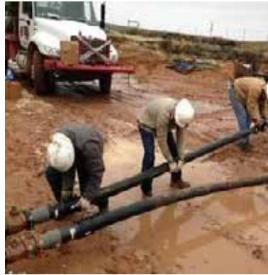
Figure 4: Example of electrofusion
