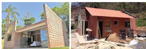
Figure 6. Model houses built using IOT in collaboration projects of UFMG with the mining companies Samarco and Gerdau. 93,94
